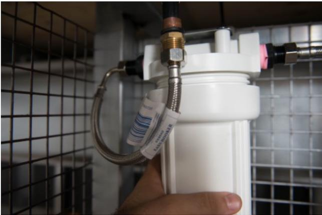
1. Twist the filter housing by hand to unscrew from base.
