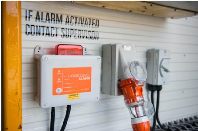
In the circumstance of a full waste tank an alert will be raised through visual red flashes from the unit as well as an audible alarm noise.
