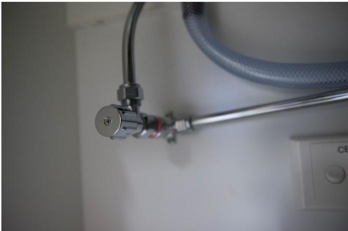
1. Open the cold water isolation valve fully on the cold water line to the boiling water unit.
