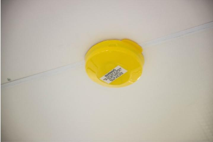
The smoke detector is located in the centre of the crib room. While the generator is running the smoke detector will use AUX power. When the generator is not operating the alarms will run on a single 12 volt battery.
