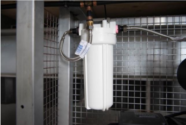
Replace every 3-6 months depending on quality of the water, standard 20 micron filter as per user manual in index section.
