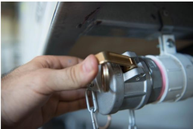
2. Access the pump out point by releasing the latches located either side of the 50mm cam lock fitting cap.
