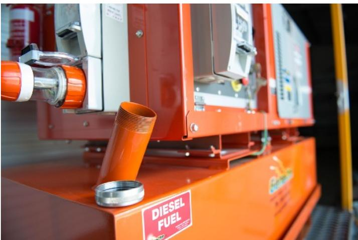
3. Fill the tank with Diesel fuel only. When finished ensure the cap is screwed back on before starting back up.
