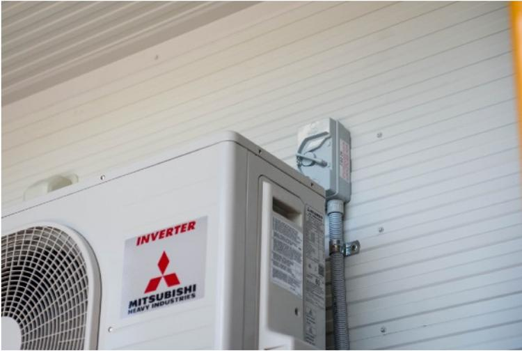
1. To use the aircon ensure the isolator switch is turned to the on position, this can be found above the generator on the front exterior of the mobile crib room.
