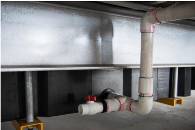
4. There is also a manual valve for waste water drainage closer to the tank. When not being used ensure that this valve is closed shut (as pictured).
