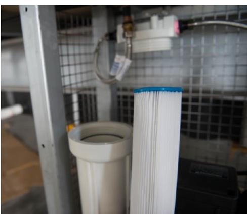
3. Remove the old filter by pulling it out and install a new one. Simply reverse the above
