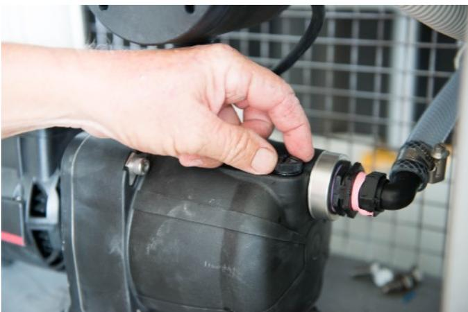
3. Locate the priming cap on the top right side of the pump and unscrew it.
