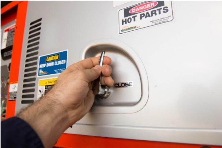
1. Checking the oil should only be performed **while the engine is cool** so there is no risk of touching hot engine machinery. Open the generator door by first twisting it 90 degrees to the right and then pulling.
