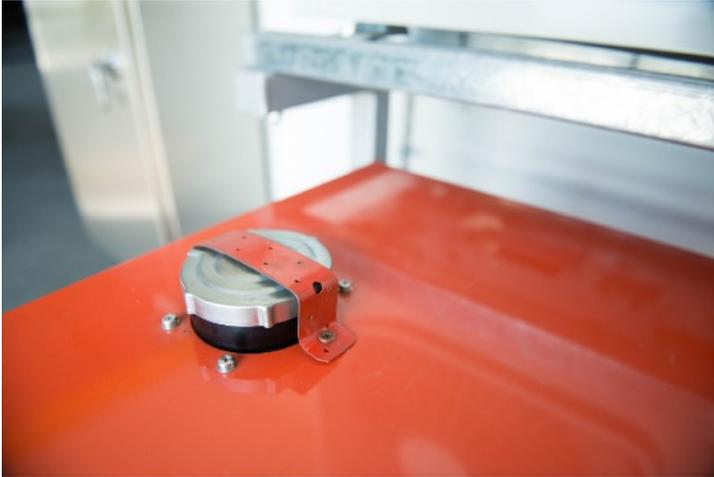
1. The generators top cap is locked shut as it should be filled up from the **230L fuel tank** below.
