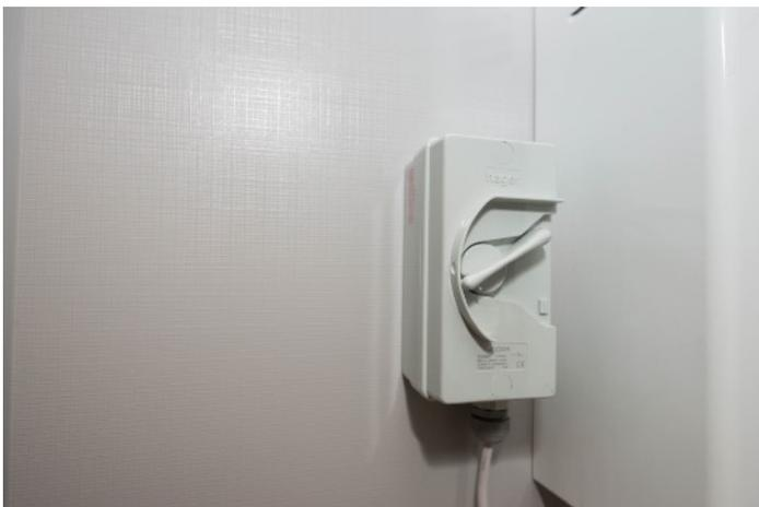
2. Switch on the electrical supply at the isolating with to the boiling water unit.
