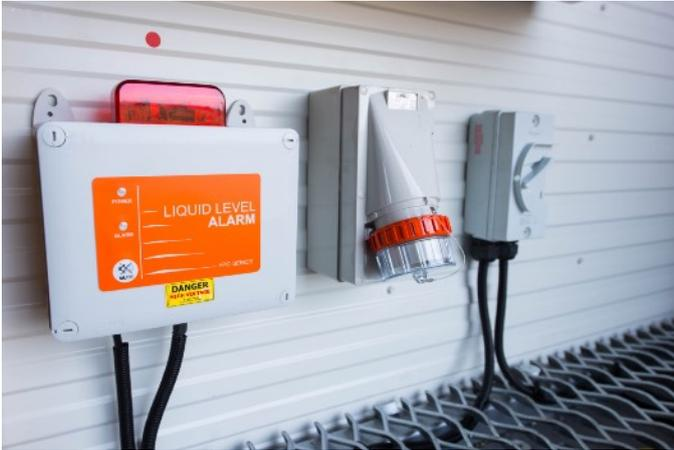
1. Locate and ensure the isolation switch is turned off while you prime. The isolation switch can be found next to the waste water liquid level alarm as pictured here on the right.
